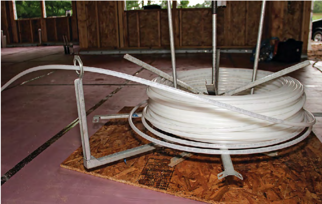
Wirubo hePEX tubing coming off the reel for the radiant heating system.
