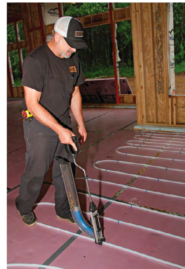
Justin Johnson used a Uponor PEX Foam Stapler to manually set the loops and secure them in place, speeding up the installation process.
