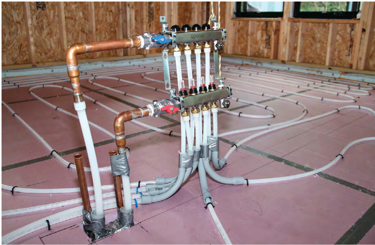
The manifold in zone four provides radiant heating and maximizing comfort in the dinette, kitchen, foyer, office, and great room.
