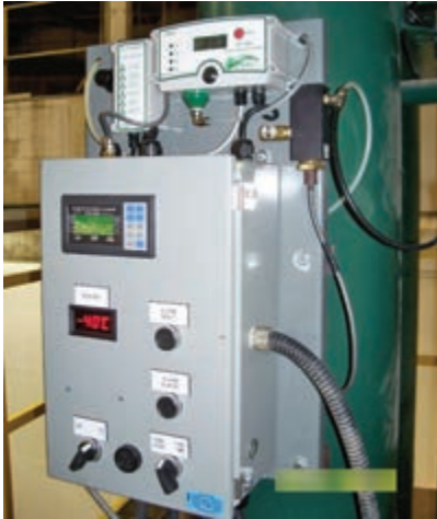
Figure 4. Dewpoint control reduced the operating cost of this breathing air purifier.
