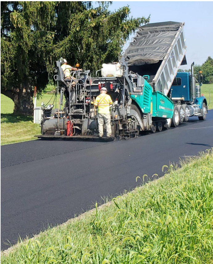
High RAP mix is shown being placed on a section of Ohio's State Road 664.
